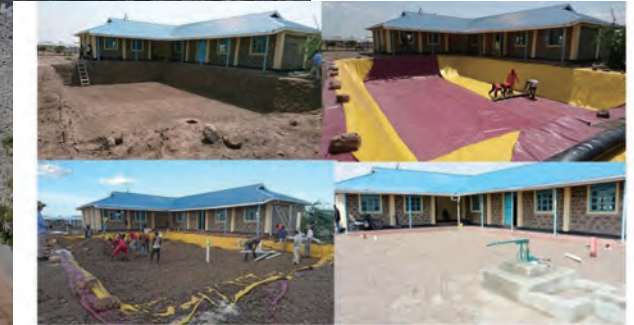
Underground rainwater harvesting tank in process at Kakobanyi settlement, Kenya
